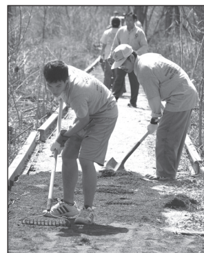
Students resurfacing a Rail Trail walking path
